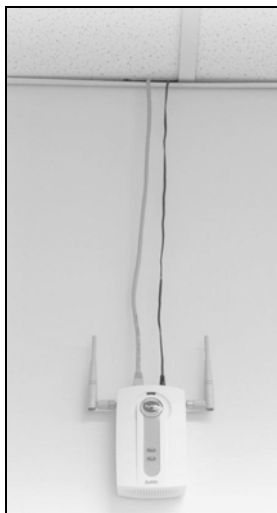
Diagram 3 Run the Cables Upward
